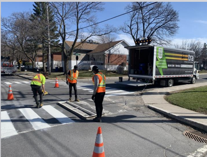
Application manuelle aux intersections
